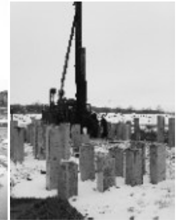
Works on Paper Factory №3 at NPPM
